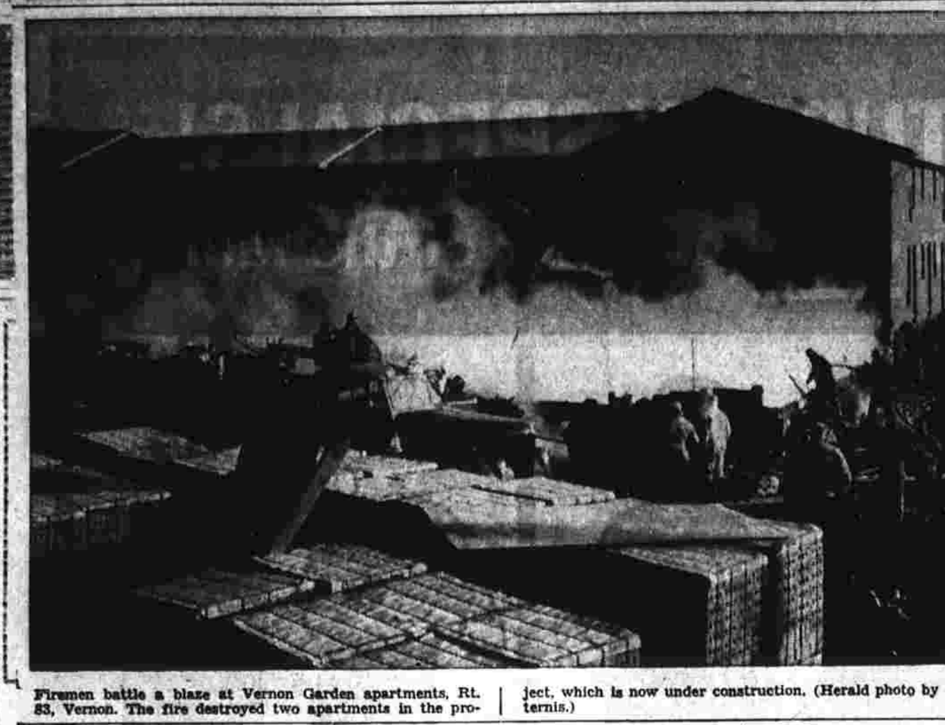
Firemen battle a blaze at Vernon Garden apartments, Rt. 83, Vernon. The fire destroyed two apartments in the project, which is now under construction. (Herald photo by S. Termini.)
